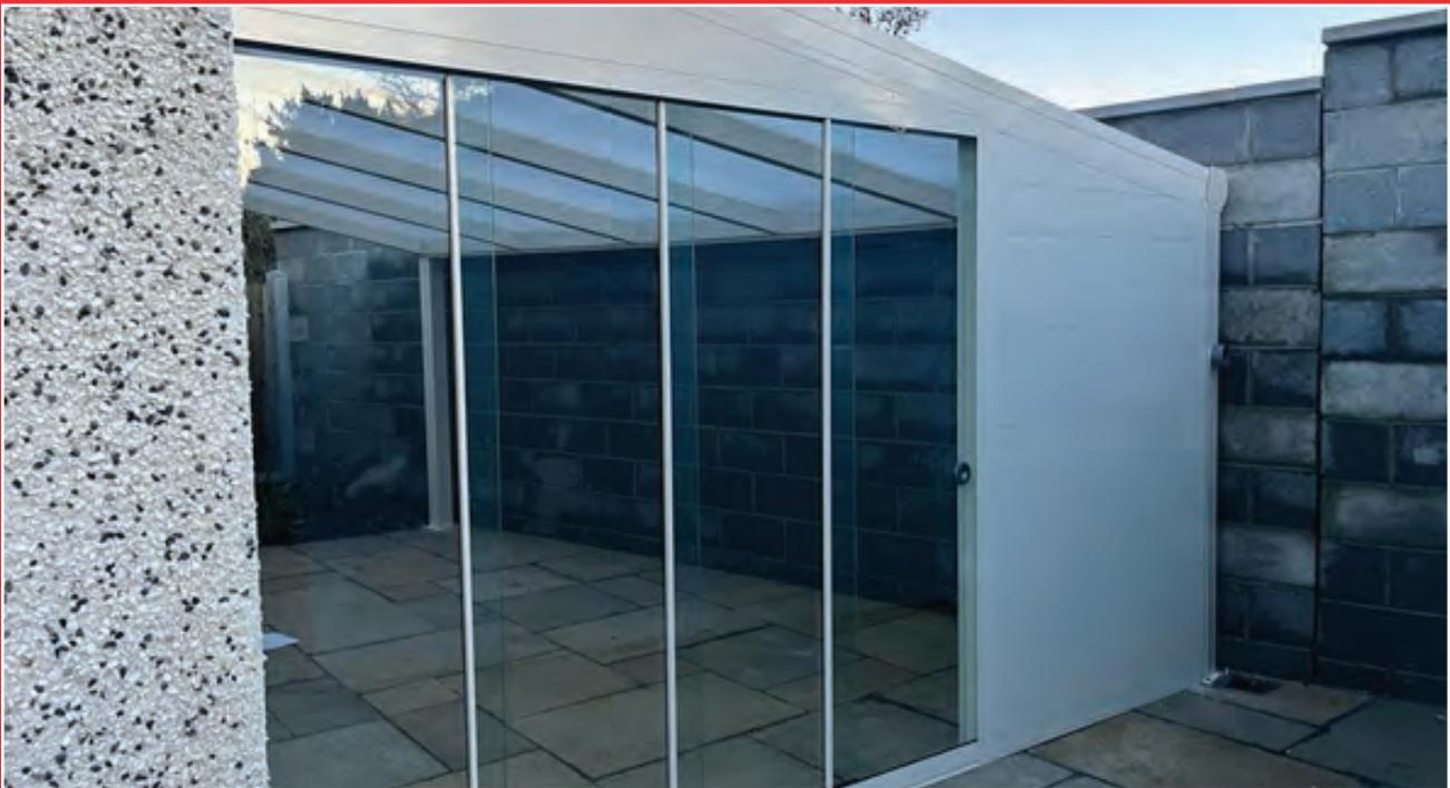
Here the "walk-in" height at the gutter is 1.8m. This 3.7m wide sidewall consists of a 2.5m wide Sliding Glass Panel set (2m high) and a 1.2m
