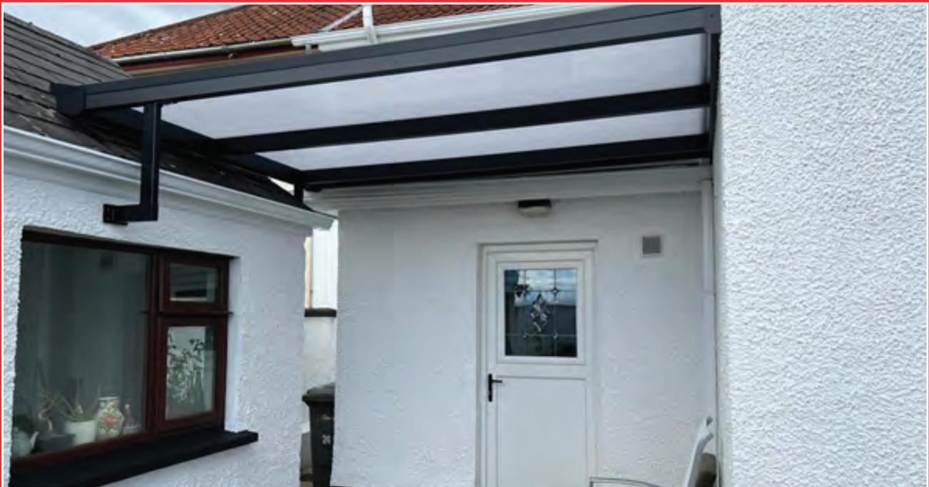
In most cases, our verandas are fitted onto your building, where the veranda backplate abutts onto your house wall and the lower front end of the veranda (where the veranda gutter is) is
