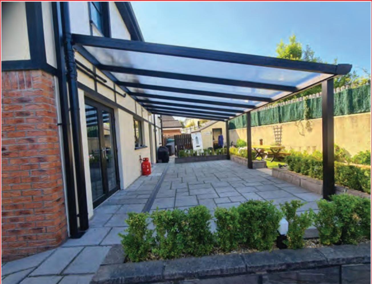
In their simplest form, our verandas are open sided (open on 3 sides) , consisting of a roof abutted onto a house wall, and projecting up to 6m out from the building. A reinforced gutter at
