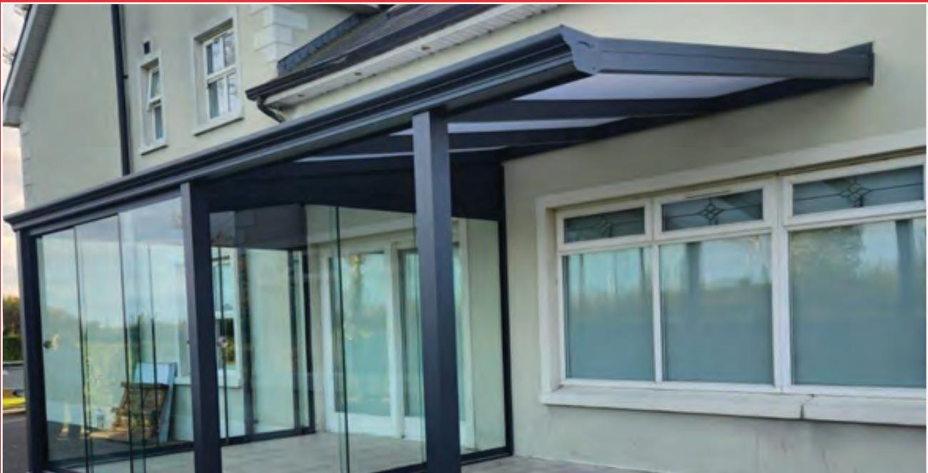
In most cases , the veranda front roof support posts are positioned at both front corners. The total number of front support posts fitted will depend upon the length of the veranda. In this case ,one of the front corner support posts is
