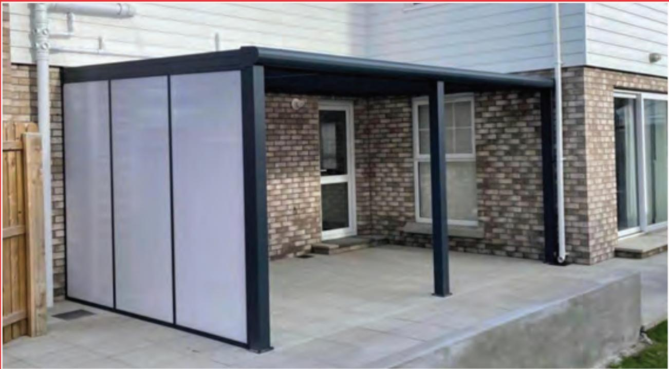
This veranda is fitted in a corner and has one of its ends fitted with polycarbonate panels. In this case it is Opal (opaque) Polycarbonate , but
