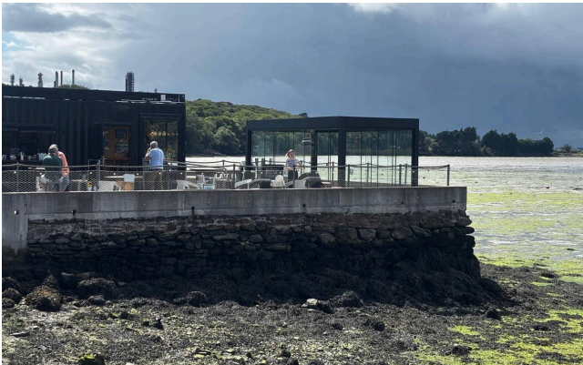
Corkbeg Coffee, Whitegate, Co. Cork. A glass room on the shore wall.
